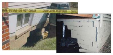
Rapidly rising floodwater can put extreme pressure on the foundation walls causing improperly vented structures to buckle and collapse. Smart Vents quickly and efficiently equalize the pressure and minimize damage.
