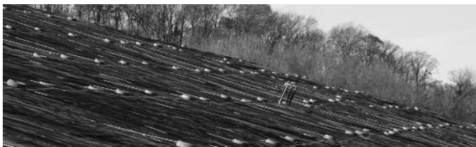
Temporary Rain Shed Cover
